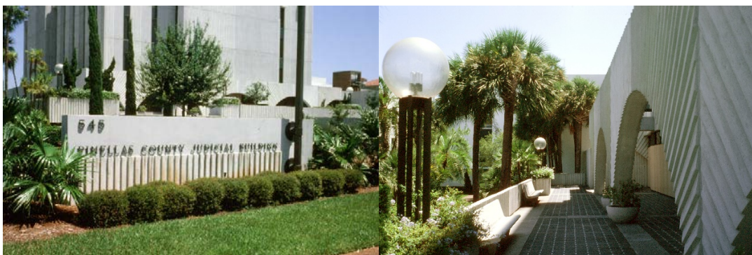
1970's building sign, open arches (later partially enclosed) - photos from Glenn Johnson's files
