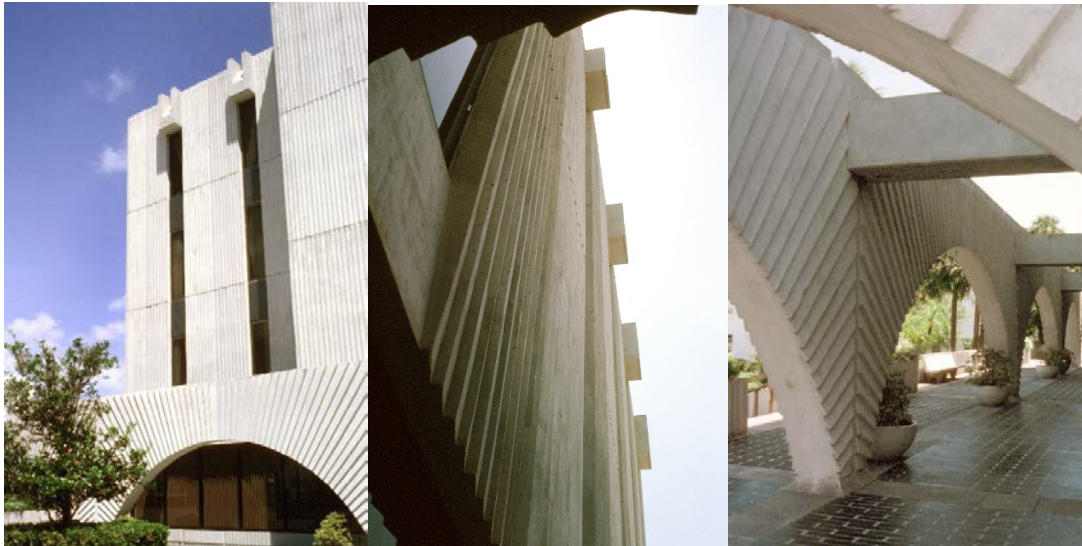
Arches filled with Styrofoam to reduce weight, rough sawn lumber in concrete forms for texture
