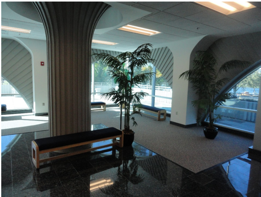
Interior of addition enclosing the columns up to the arches – author’s photo
